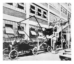
component onto the unit, till it rolled off the line fully assembled. Yet an even more startling innovation was required in order for assembly lines to function. What truly allowed Ford to leapfrog the competition was the idea of interchangeable parts.
